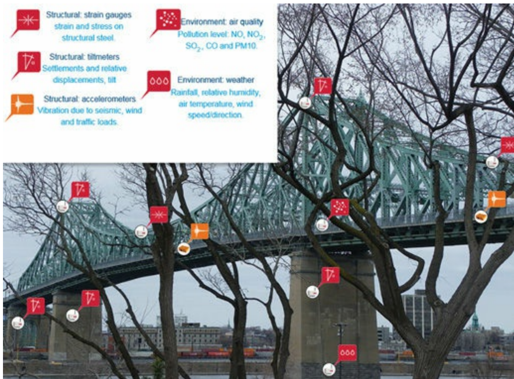
Figure 13-2 Smart Objects Monitoring a Bridge
