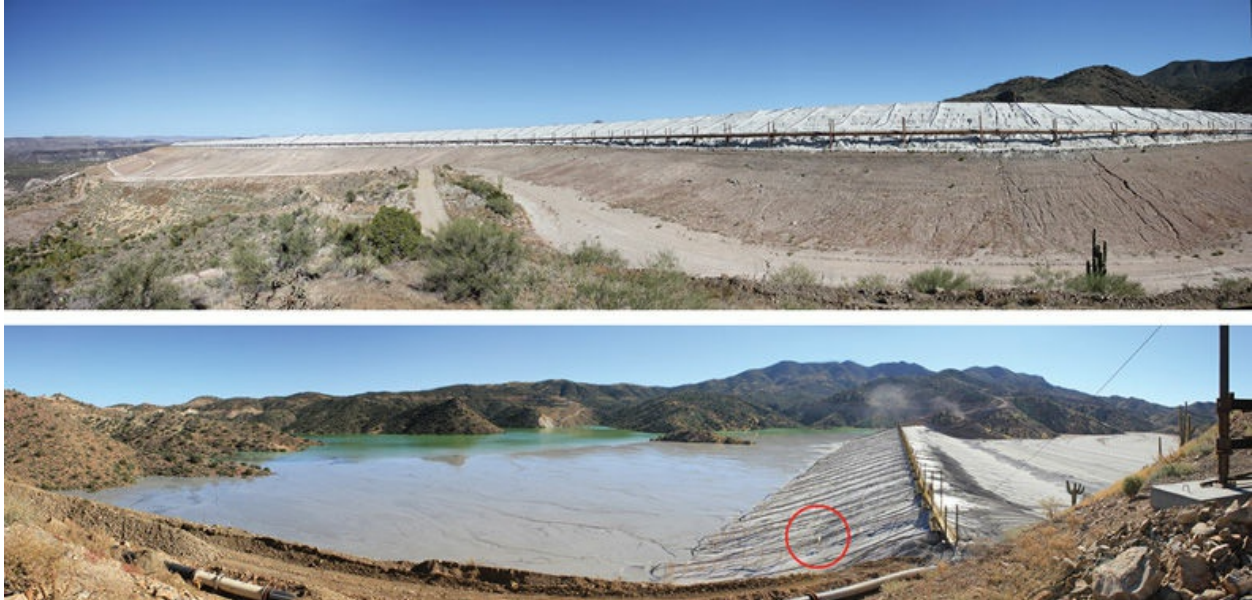
Figure 14-10 View of an Earthen Dam from the Outside (top) and Tailing Pond with an Earthen Dam (bottom)
